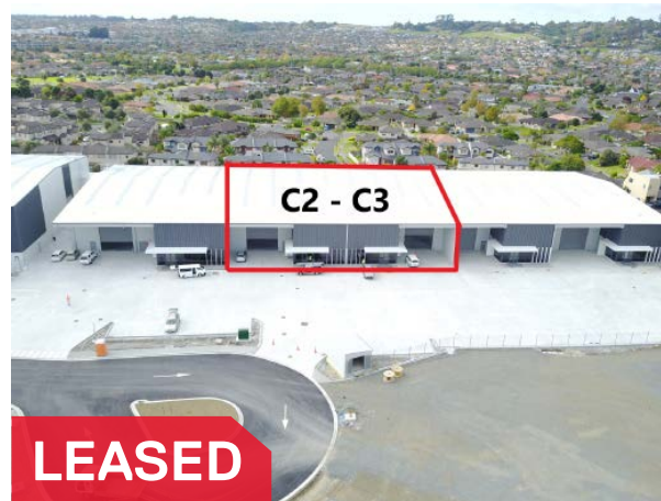
Unit C2 & C3, 27 Smales Road, East Tamaki Annual Rent | $295,677 Building Area | 1,363m 2
