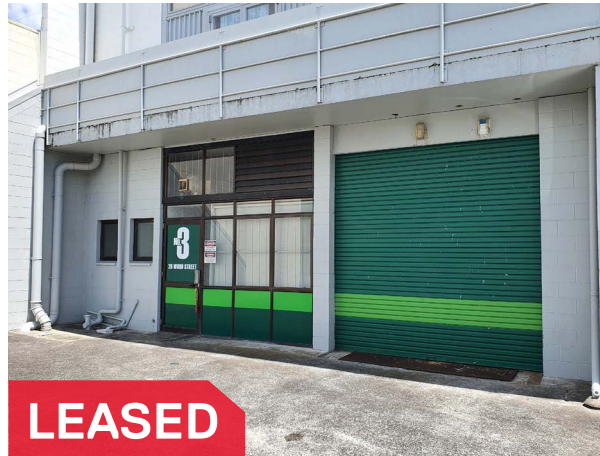
Unit 3, 26 Wood Street, Papakura Annual Rent | $40,000 Building Area | 198m 2
