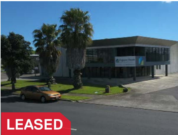
38A Greenmount Drive, East Tamaki Annual Rent | $151,555 Building Area | 850m 2
